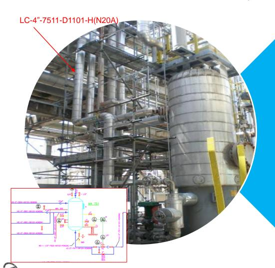
To carry out visual inspection for the designated line. The inspector is responsible to physically visualize the line against the as built isometric drawing.
