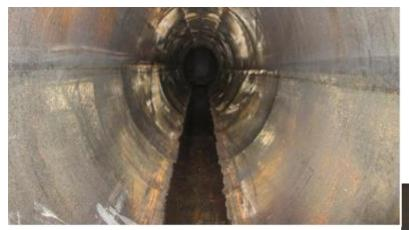
Internal surface of the shell w/o signs of corrosion pits
