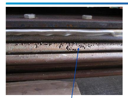
Slightly deep corrosion pits
