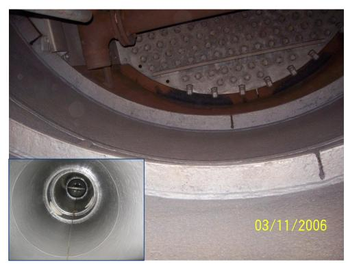
The acid washing process at elevated temperature led to severe pitting within the tower and significant loss of wall thickness adjacent to tray support rings. High Temperature repair compound used to restore wall thickness then acid resistant lining applied to resist operating conditions at 95C - Inspected in Year 2011 and in good condition.
