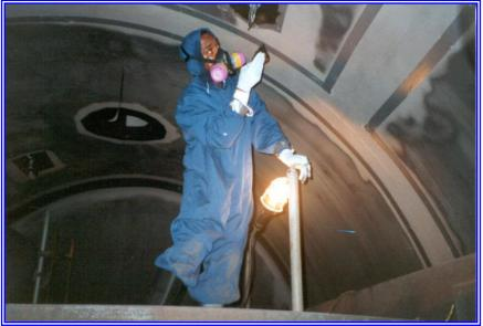
Protection of weld areas subject to stress corrosion cracking at elevated temperatures due to the presence of H2S. Weld areas only protected using high temperature Hybrid Epoxy Novolac lining system with operating temperature in excess of 150C
