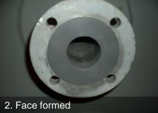
Flange face forming and small bore nozzle protection, applied in 2009, inspected in 2013.
