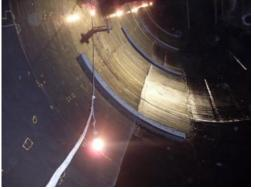
4 pressure vessels - in-service temperatures of up to 180°C. Adjacent flange faces and nozzles also required corrosion protection. Inspected in 2013, all in perfect condition.
