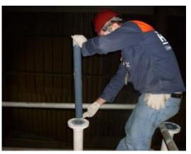
Belzona nozzle inserts bonded into small bore nozzles, protect against corrosion and erosion
