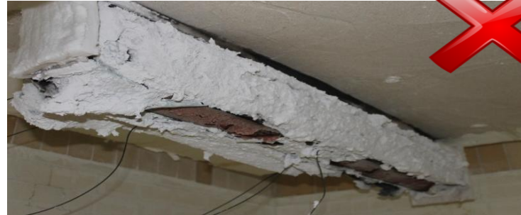
Bad stickability: lack of adhesion steel-primer causing char detachment
