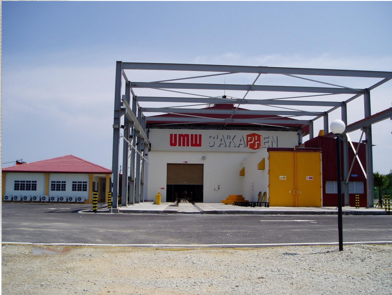
coating Workshop in TELUK KALONG, Malaysia of our Licensee UMW SAEKAPHEN COATING SDN BHD
