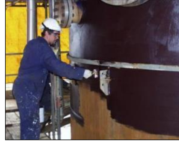
Application of Heat Activated Coating System using rollers and brushes
