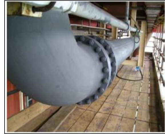
Heat Activated Composite wrapping and coating carried out on-line
