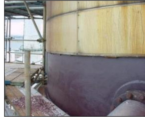
Application of Heat Activated Coating System using rollers and brushes
