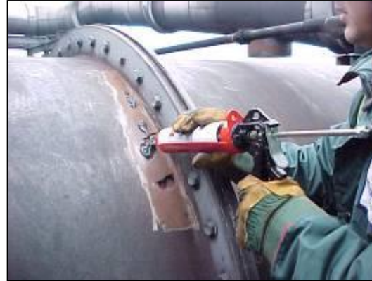
Filling of Pitting Corrosion
