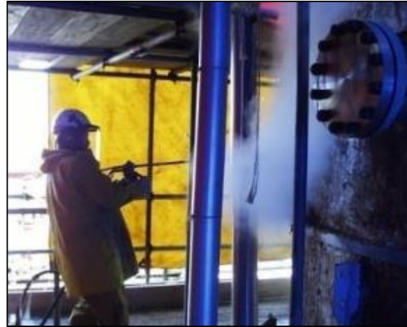
Surface Preparation Carried out Using High Pressure Water Jetting
