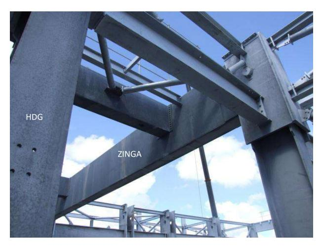
20-ton box-beams used to build Runcorn Power Station in UK Combination of HDG and ZINGA on same project!
