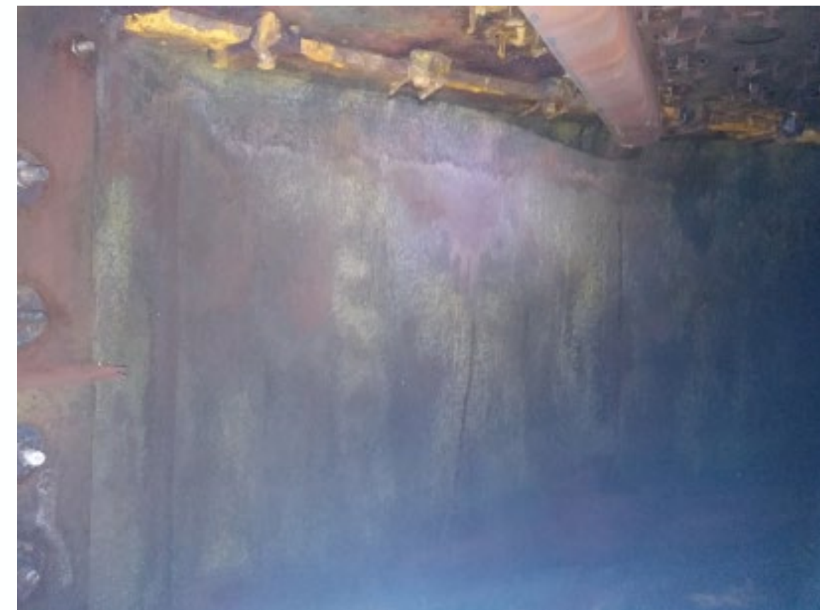
Inspected again in July 2023.
