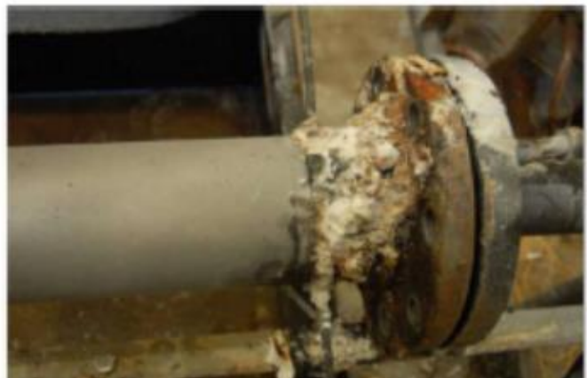
3B(non-coated) Negligible Corrosion
