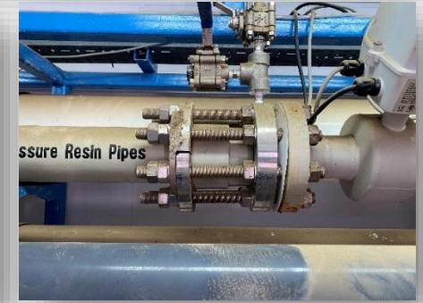
Coupling and flange joints of HPRP
