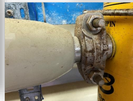
Coupling and flange joints of HPRP
