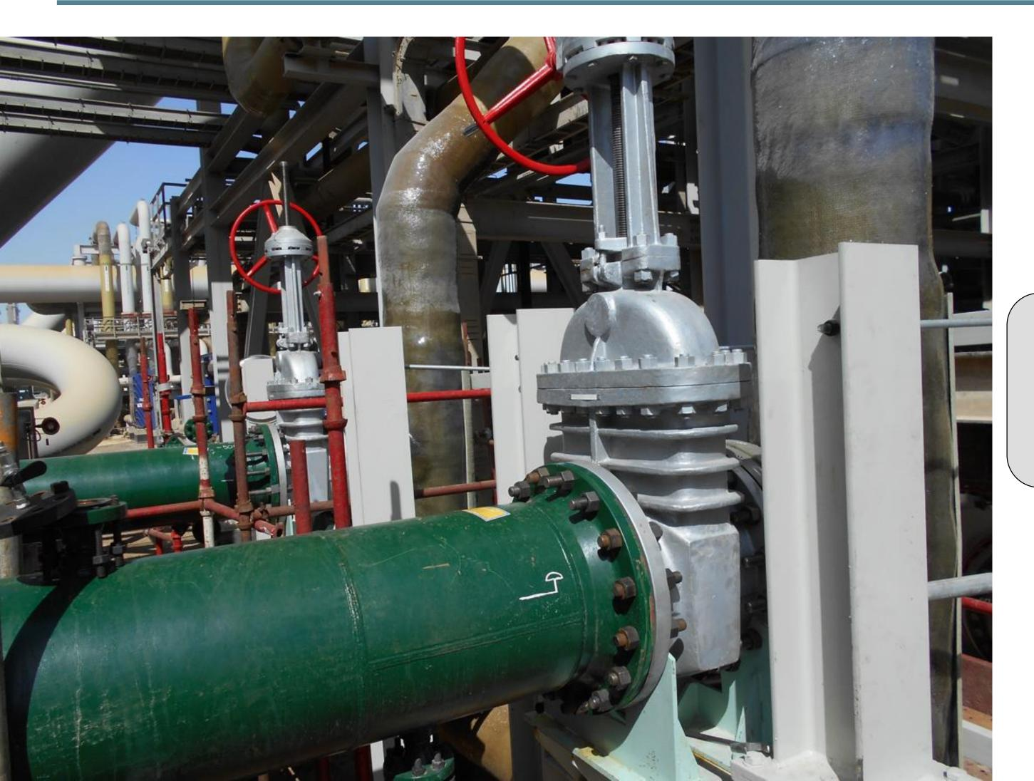
Sleeve Installation & connection with Gate valve/Hot tapping/Isolation Machine setup
