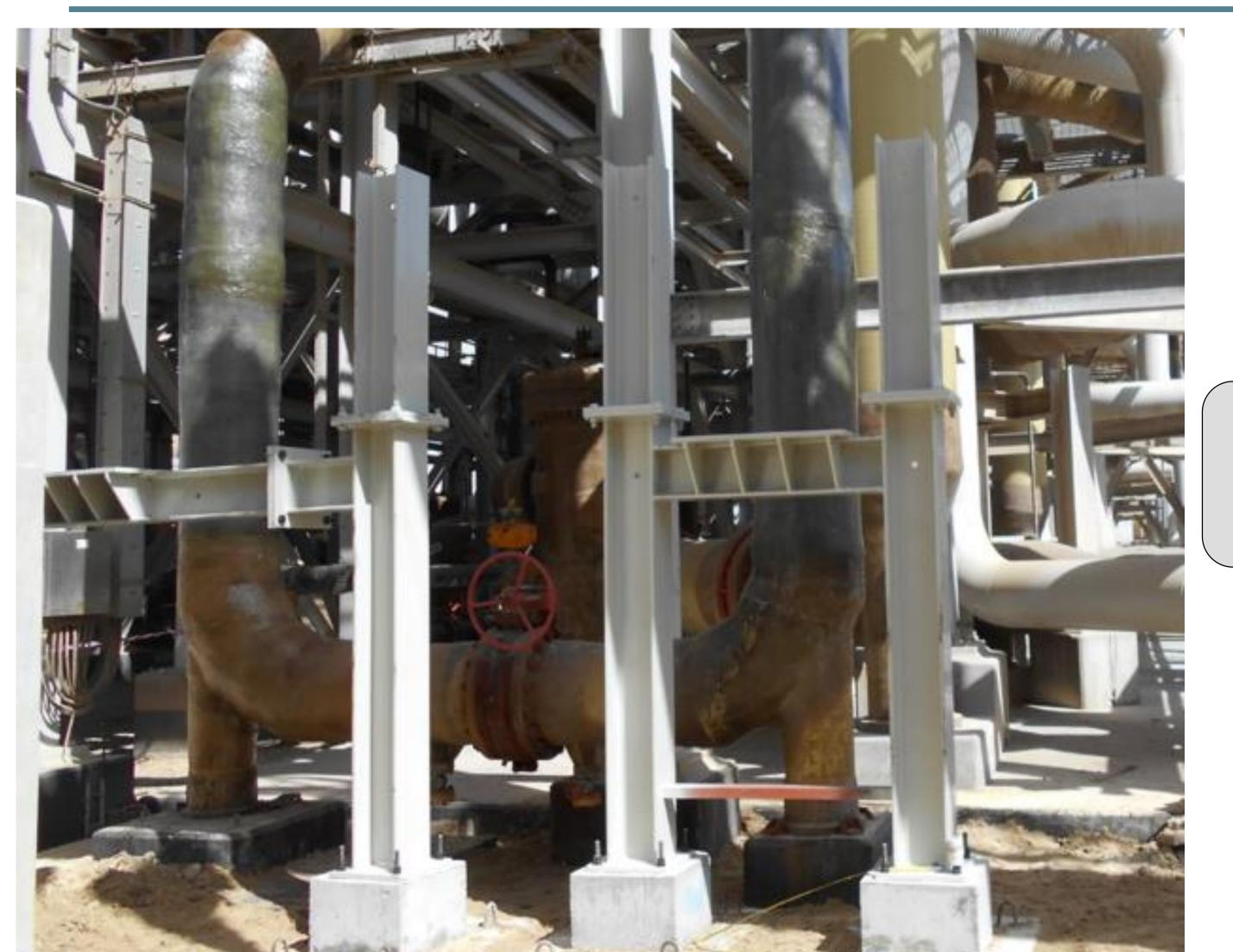
Local Reinforcement and Support Erection for Gate Valve.
